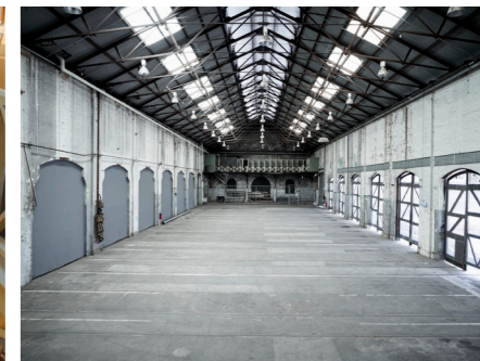
Carriage works - Bay 22-24
